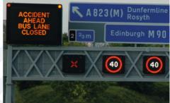
In emergency situations, the motorway signal over the bus lane is used to advise bus drivers that the bus lane is closed – a red  $\mathbf{X}$  signal is displayed over the bus lane and the variable message sign reinforces this.
