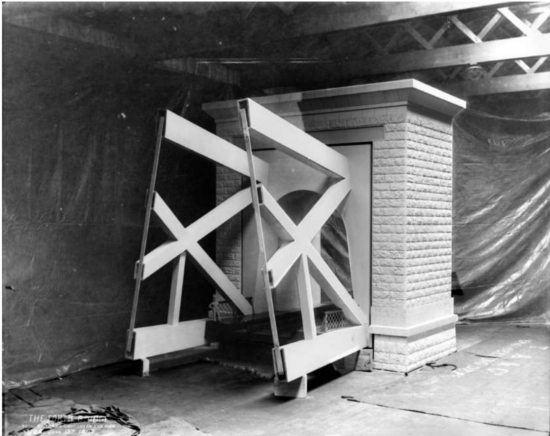
Crown copyright, National Records of Scotland, BR/FOR/4/34/124, Model of top of cantilever end pier, showing connection with the cantilever, 13 Jun e1887;
