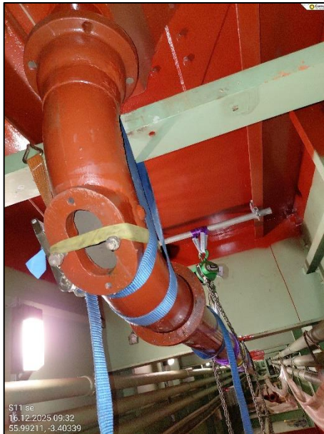
Reinstall of primed downpipes commenced
