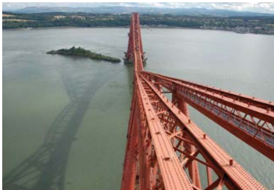
The Inchgarvie tower and island, with the Lothian coastline in the background, August 2012. (© Crown Copyright, reproduced courtesy of Historic Scotland. www.historicscotlandimages.gov.uk , Miles Oglethorpe, DSC_7935)
