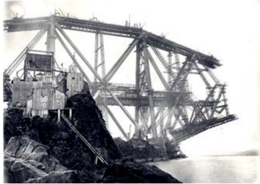
Left: The Inchgarvie tower taking shape in 1888. (© Crown Copyright, National Records of Scotland, BR/FOR/4/34/436)
