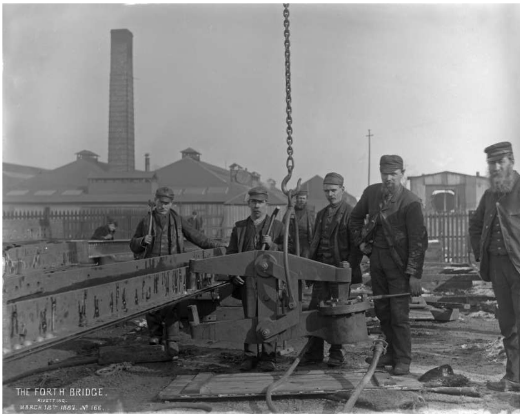
Crown copyright, National Records of Scotland, BR/FOR/4/34/116, Riveters posed with a pneumatic riveting machine on the drill roads, 12 Mar 1887
