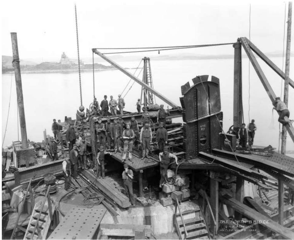
Crown copyright, National Records of Scotland, BR/FOR/4/34/318, Queensferry north east cantilever bedplate, 9 Jul 1886
