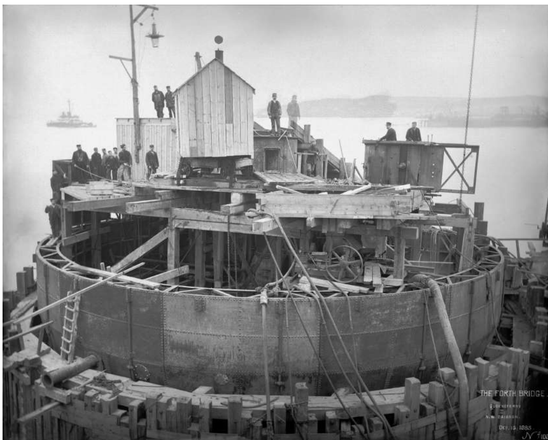
Crown copyright, National Records of Scotland, BR/FOR/4/34/176, Queensferry north west caisson, 15 Dec 1885
