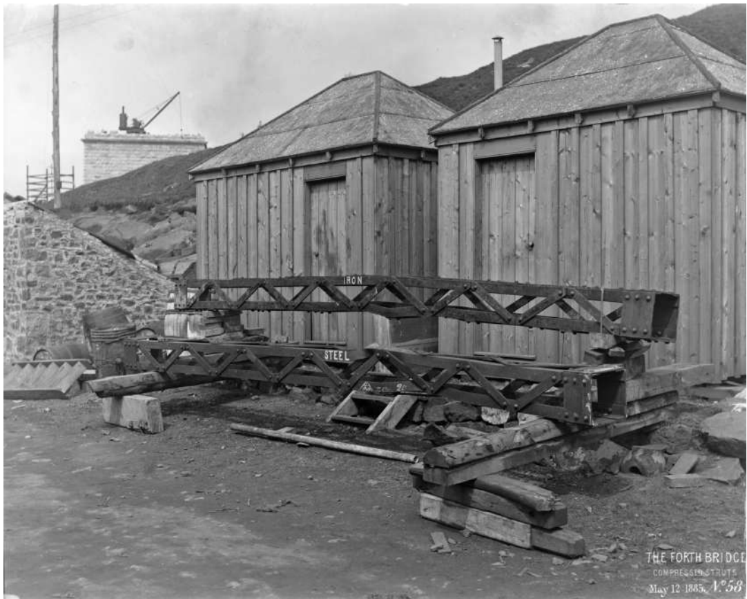
Crown copyright, National Records of Scotland, BR/FOR/4/34/123, Compressed struts, one labelled iron, one labelled steel (possibly for testing the metal), in front of two workers' sheds, 12 May 1885
